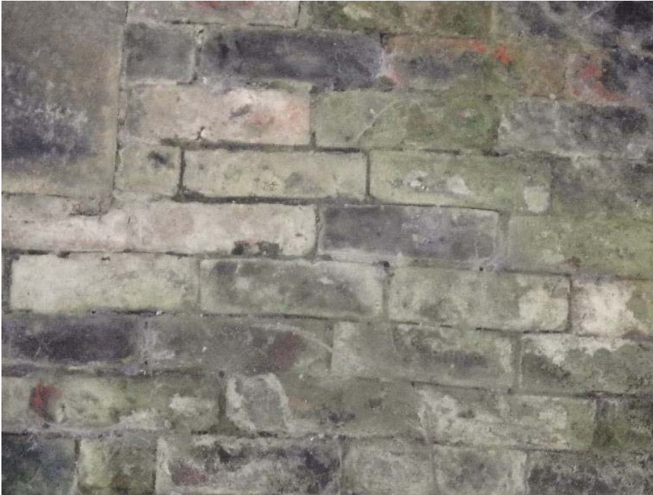
9) Movement to brickwork in southeast haunch
