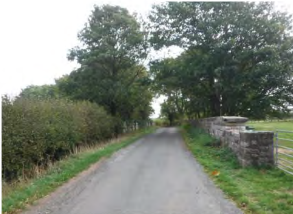
Photo No: 8 – View: Across Structure.
