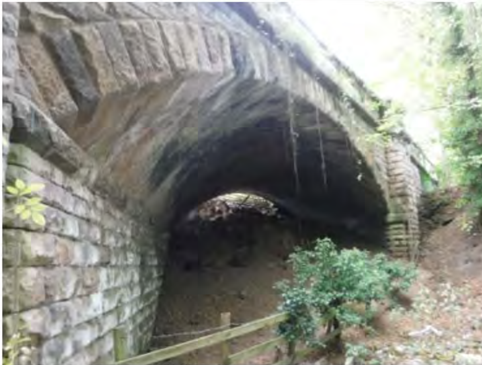
Photo No: 7 – Arch ring soffit: View.
